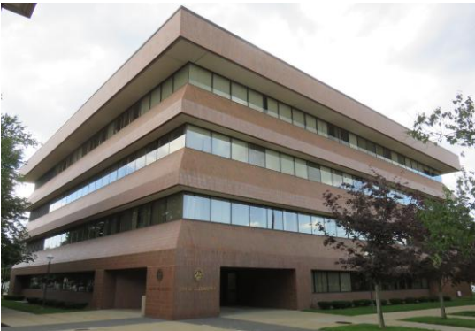
Midland County Services Building
